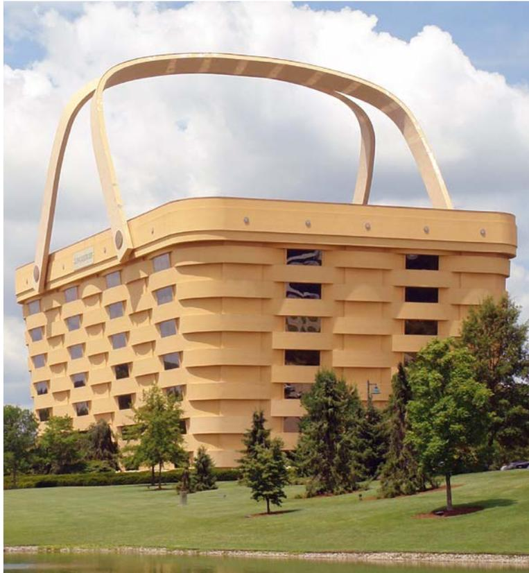
The giant handles of this basket alone weigh almost 150 tons. The handles are heated to keep ice from forming.
